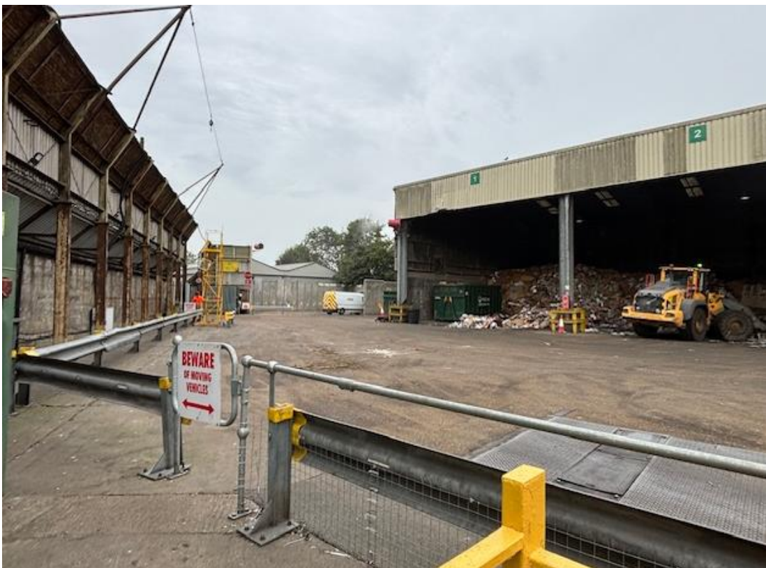
Figure 7 – Facing north west
