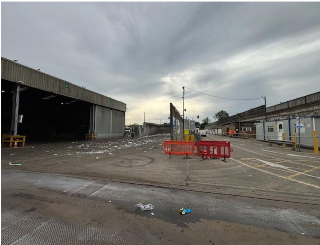
Figure 9 – Facing south east
